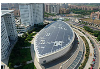
The photovoltaic installation financed by BBVA on the Valencia Congress Hall
