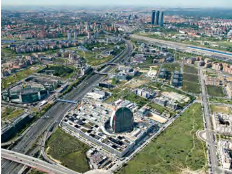
Since the location offered no points of urban reference, we developed the campus from inside out as a horizontal fabric, while ensuring that it can be seen from the motorway
